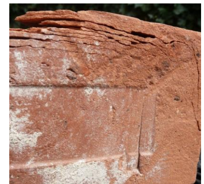
DELAMINATION
