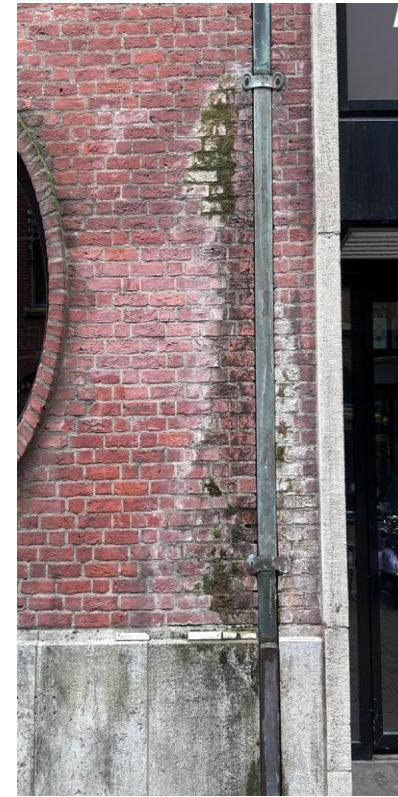
INFILTRATION & LEAKAGE
