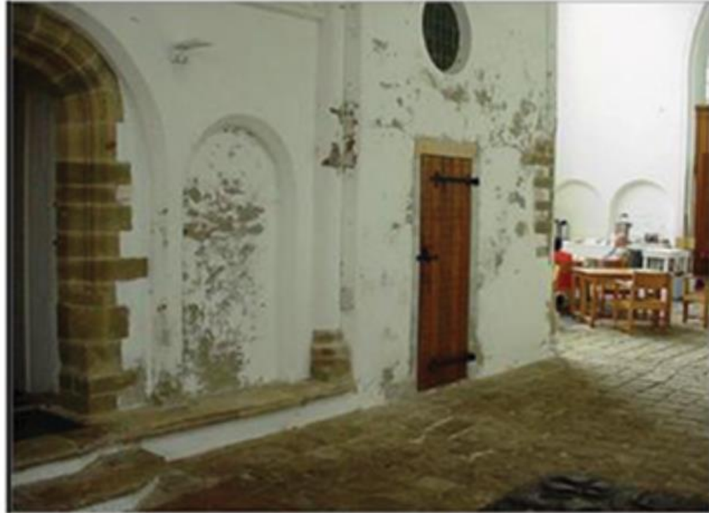
Development of salt crystallization damage over a period of 5 years (Van Hees et al., 2020)
