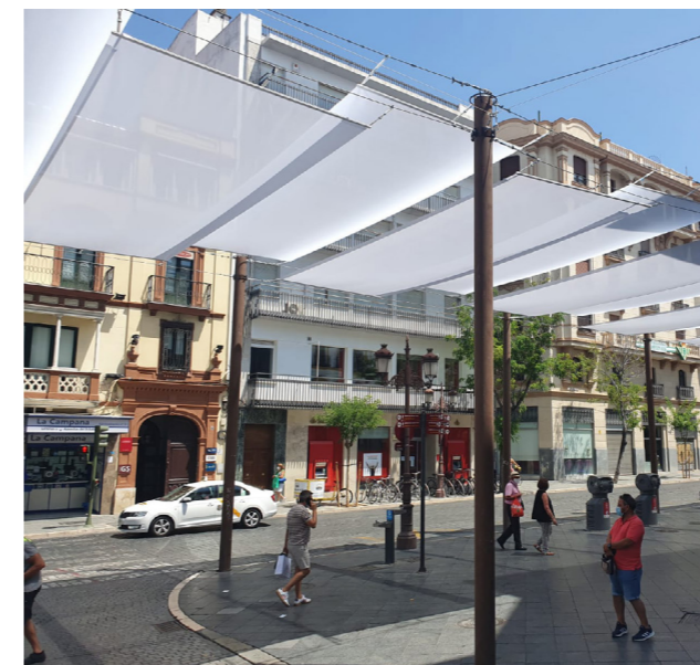
Figure 08. [Heat] Using Overhangs to block sunlight, Seville Spain. (Centro Historico, 2022)
