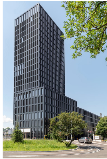
Figure 63: BIPV façade (rainscreen). Basel, Switzerland. Source: SOLAR (2022)
