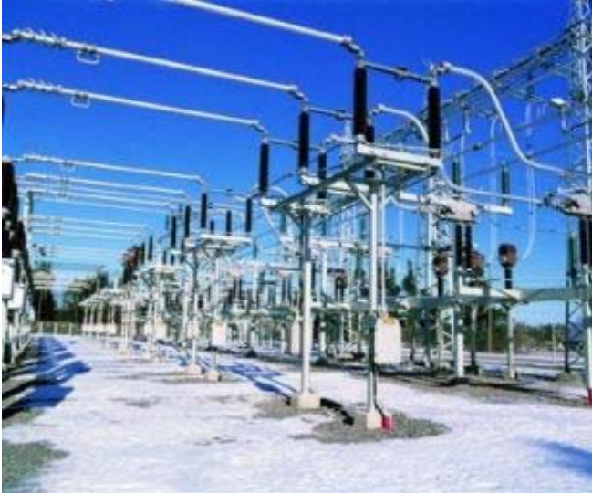
Figure 1.3 centre break disconnector in closed position [ Hapam website].
