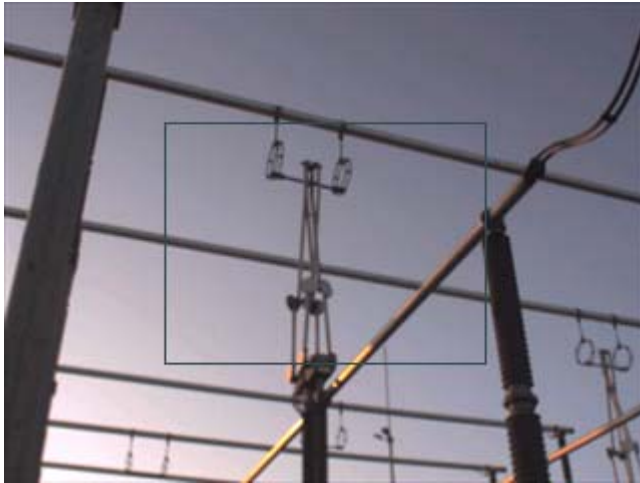
Figure 1.5 pantograph disconnecter in closed position
