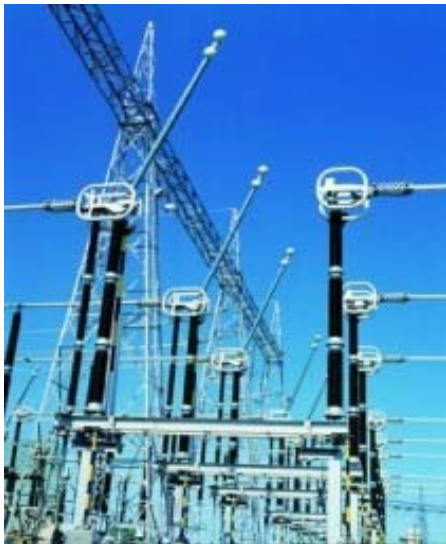
Figure 1.6 Vertical break disconnecter in open position [ Hapam website].
