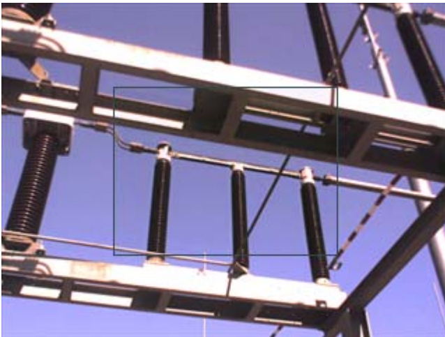
Figure 1.4 double break disconnector in closed position
