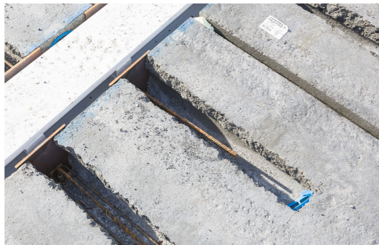
Figure 10: Top and bottom: Demountable channel plate floors (cepezed, 2024)
