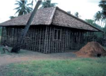
fig. 64 Swahili house in Bagamoyo under construction (1985) see also figs. 4 and 9
