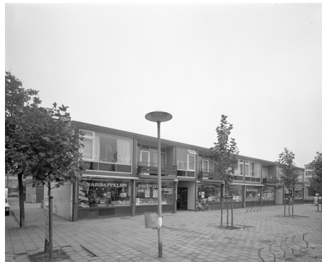
*1983 two-storey residential-commercial housing block
