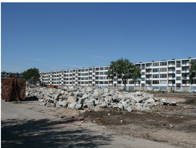
Figure 26 Demolition of the Intervam flat in Donaudreef. (Photo link: http://mapio.net/sl42073773/ )
