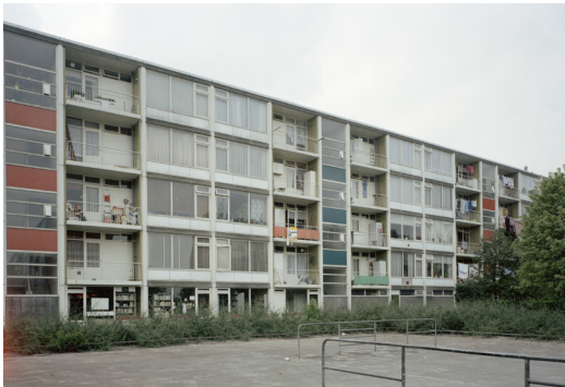
*1984 wooden window frames of the facade (before the renovation)
