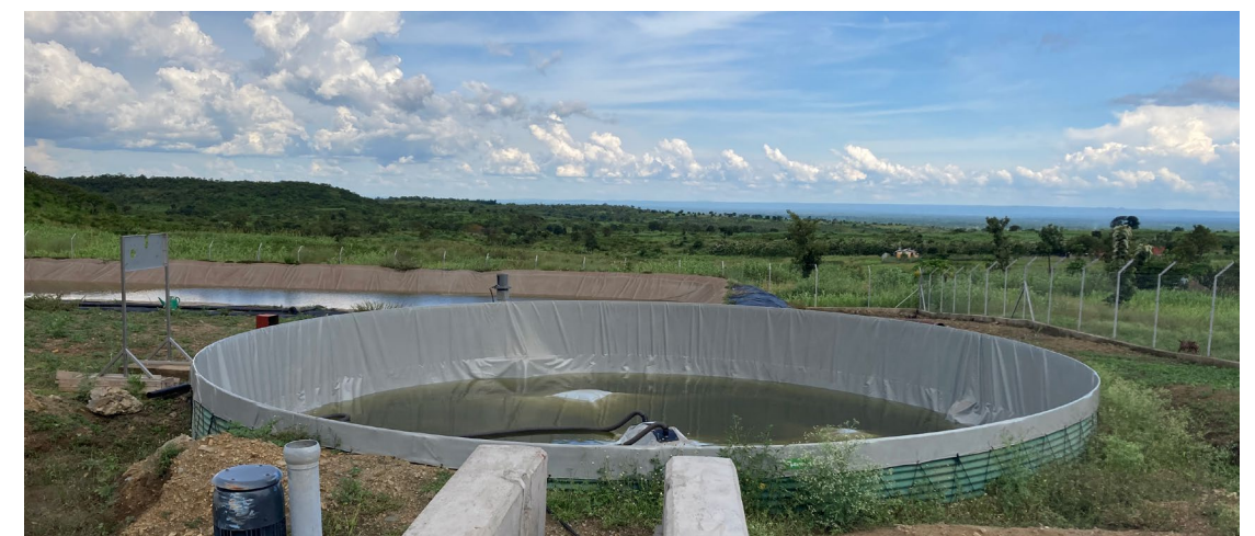
Fig. 1.7 | The biodigester set up by the Waste to Clean Air project (under construction)
