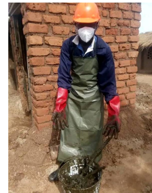
Fig. 2.32 | Rehydrating sludge in an unlined pit latrine causes direct contact between the worker and fecal matter
