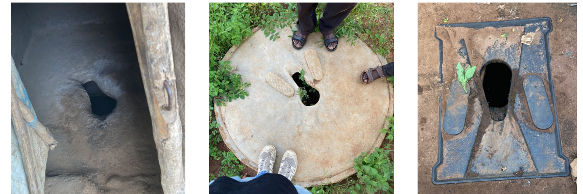
Fig. 2.15 | Latrine 'slabs' from left to right: sticks & mud, concrete, plastic
