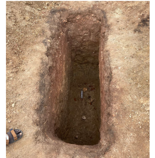
Fig. 2.14 | Excavated latrine hole
