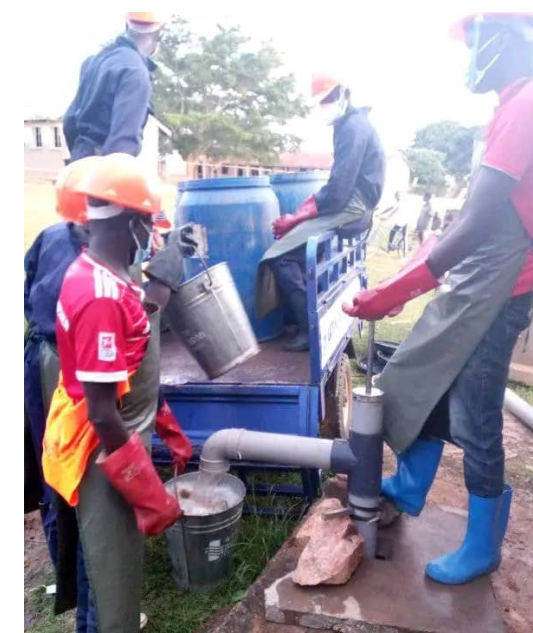
Fig. 2.31 | Operators of the gulper work directly above the fecal sludge
