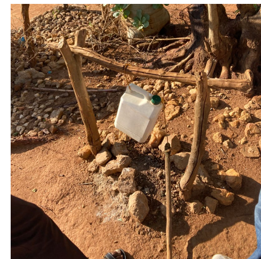
Fig. 2.21 | Handsfree hand washing facility using sticks, rope and a jerrycan
