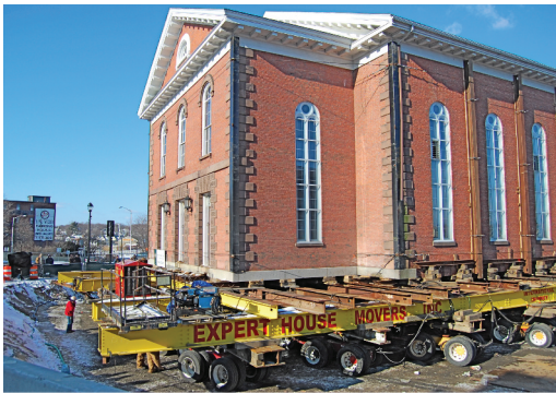
Figure 3. Large historical building relocation, 2009, Salem, Massachusetts.
