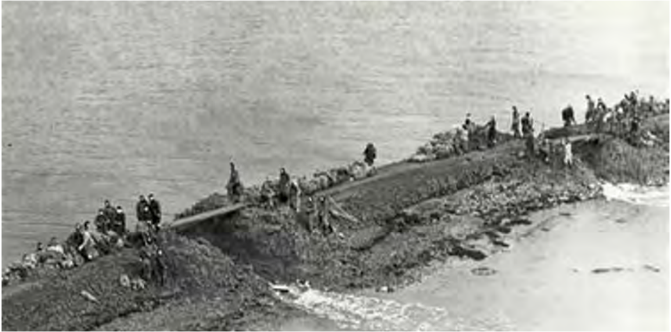
FIG. 1.12 1953 Flood in Sheppey. Flood water being drained from the land by means of cuts in the river wall near Kings Ferry Bridge. Source: https://www.kentonline.co.uk/kent/news/ .
