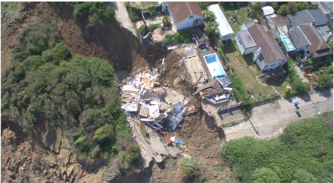
FIG. 1.13 Coastal erosion: The 'forgotten' community left to fall off a cliff. July 2020. Source: BBC news. https://www.bbc.com/news/uk-england-53367000 .
