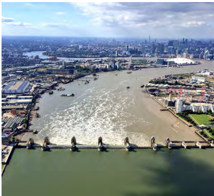
FIG. 1.14 Thames Barrier. Image source: NPAS London & South East Region.
