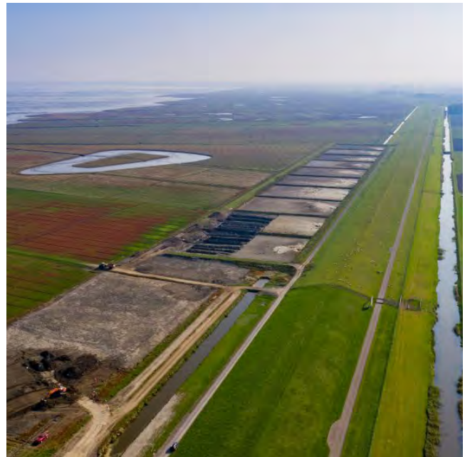
FIG. 4.4 Pilot sludge sedimentation (Image source: Eems-Dollard 2050)
