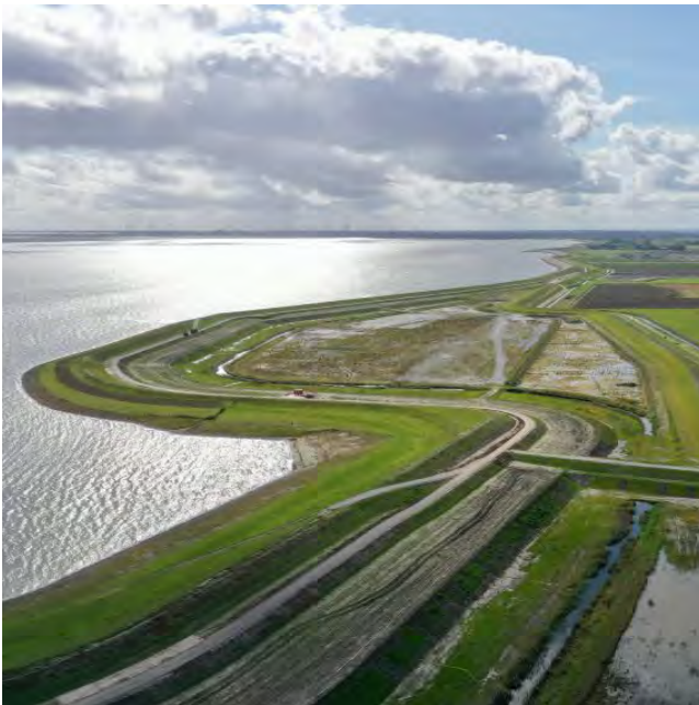
FIG. 4.3 Pilot double dike (Image source: Eems-Dollard 2050)
