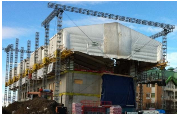
Figure 1. Overall protection of construction site (Sunderby hospital, Sweden, 2013)
