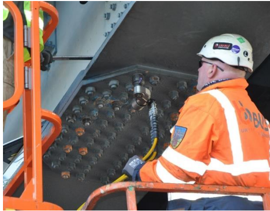
Figure 5.12: Loosening the nut with a hydraulic torque wrench
