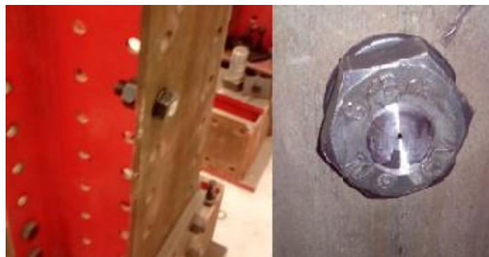
Figure 4.21: Bolt B3 with implanted strain gauge
