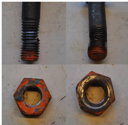
Figure 5.29: The painted extended part of the bolts below the nut
