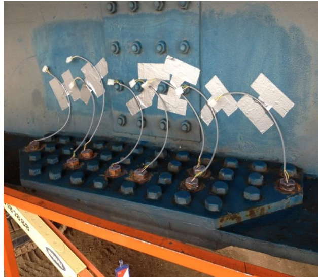
Figure 5.10: The connection after the installation of the strain gauges
