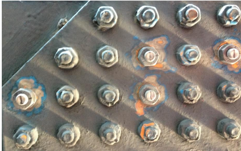
Figure 5.15: Marked nuts, bolts after the combined method was applied
