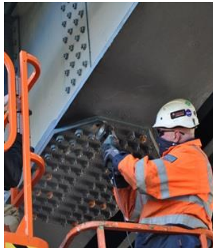
Figure 5.16: Grinding of the plate surface
