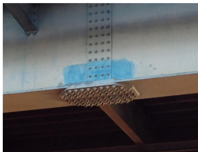
Figure 5.2: The tested connection
