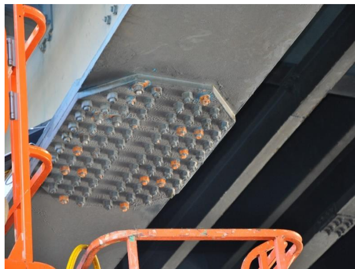
Figure 5.17: New bolt tightened on the connection
