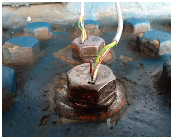
Figure 5.8: Bolts after the installation of the strain gauges
