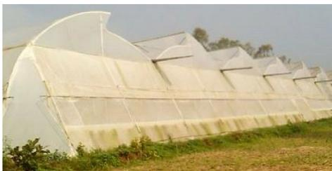
(c) Gutter Connected Greenhouse
