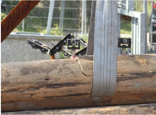
Figure 3.19, Soft shell visible during loading of pile 4 at load step 14 of 26. Soft shell ‘cracks open’.
