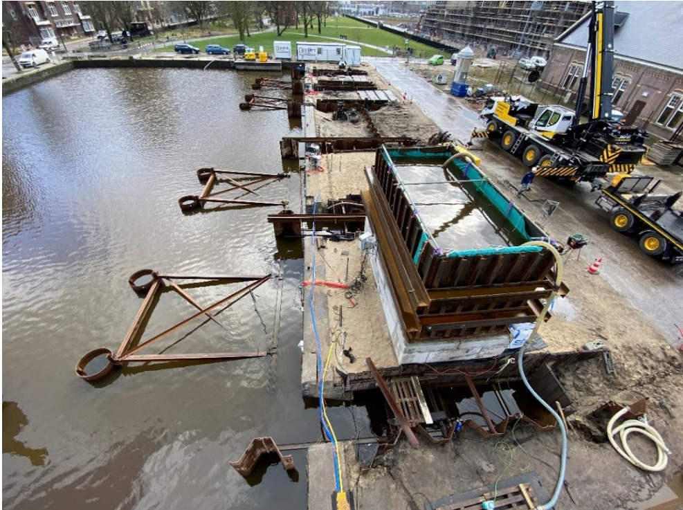
Figure 2.13, Proof load experiment on quay wall segment.
