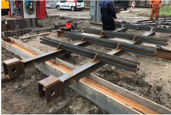
Figure 4.25, Steel frame to be installed underwater and connected with tension slings to the 3x4 pile matrix.
