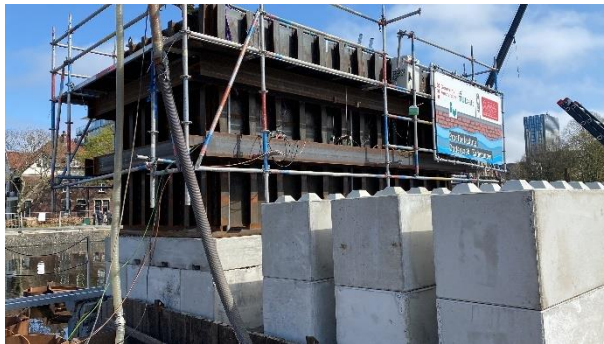
Figure 5.20, Extra ballast behind container in experiment A.II.
