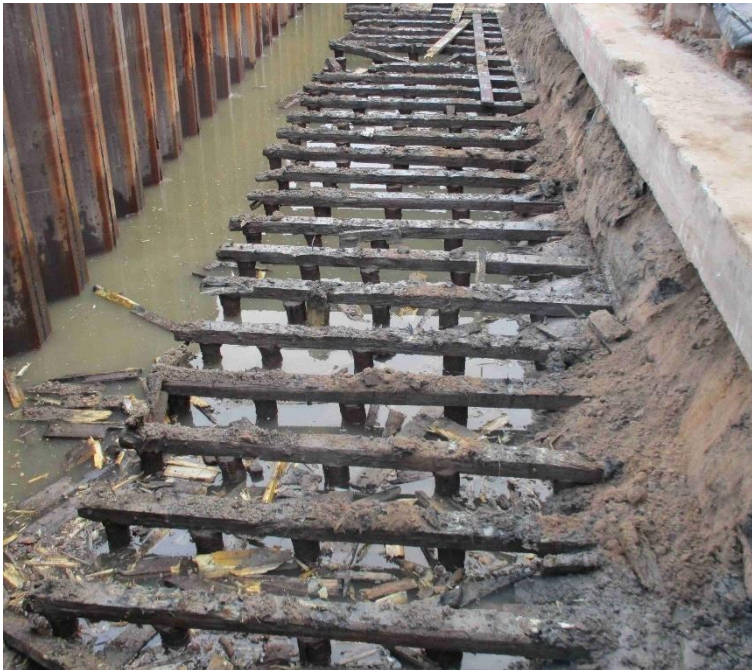
Figure 4.2, Excavated historical quay wall, 'Maaskade' in Rotterdam. Left of the pile foundation, the water is situated and right the hinterland used to be present. Photograph: Julianus, Eric. "Exposed timber pile foundation of the Maaskade". 2019. Havenbedrijf Rotterdam.
