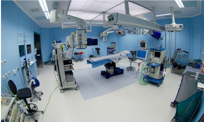
Figure 4.7: This is an OR in the RdGG. The blue rectangle on the floor marks the sterile zone. The operation table stands in the middle of this zone. When properly dressed, you may enter this zone. Other staff walks around this zone control or hand over other equipment [17].
