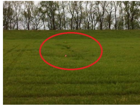
(b) Settlement due to collapsed pipe along the Mississippi, Ensley levee [USBR and USACE, 2019].
