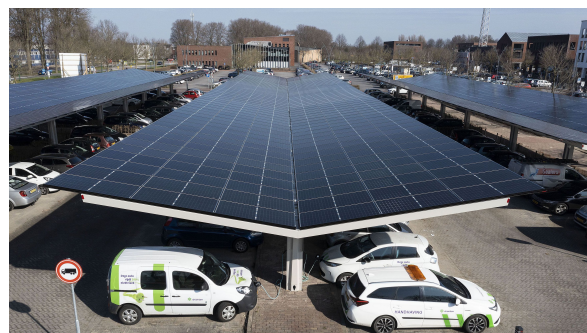
Figure 3.9: T-frame carport structure at the car park in Dronten, Source: Fotostudio Wierd
