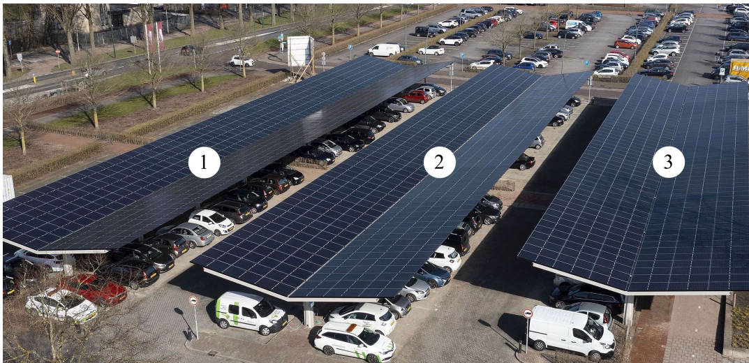
Figure 3.2: Layout of the solar car park with row numbering, Source: Fotostudio Wierd
