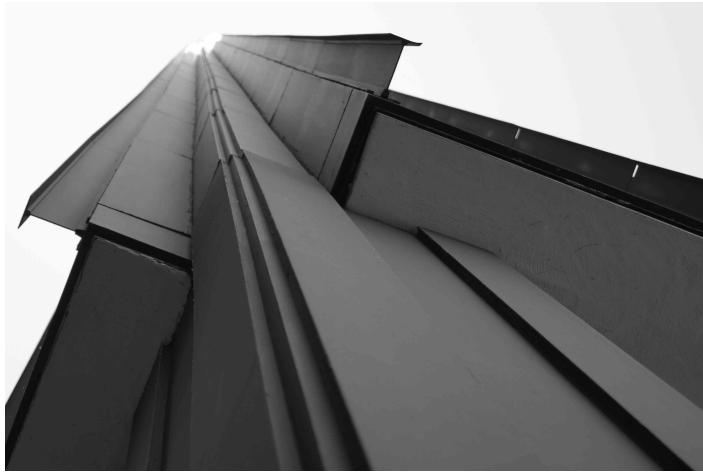
Fig. 21. (left) I-beam mullions of the Lake Shore Drive apartments. Source: https://skylinearchitecture.wordpress.com
