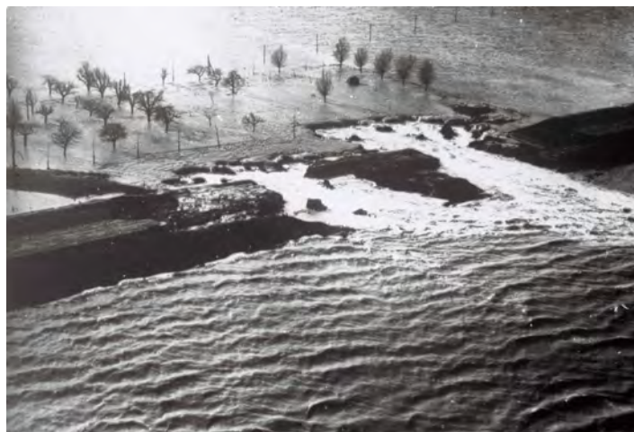
Figure 1.1: Breached dike during the flooding disaster in the Netherlands (Rijkswaterstaat, 1953)
