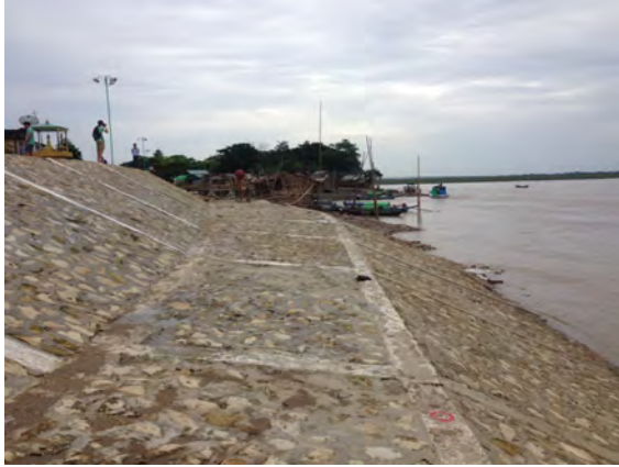
Figure 4.18: Outer slope strong dike type 1 (by Nick Stoop)
