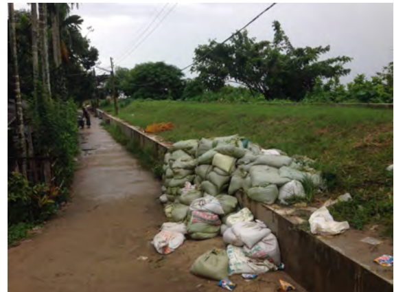
Figure 4.15: Inner slope dike (by Nick Stoop)
