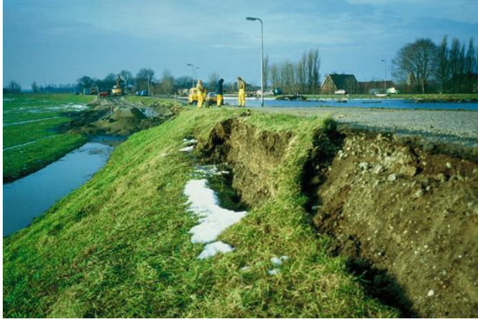
Figure 2.11: Remaining profile after first sliding in Schipluiden (South Holland) (Den Haan et al., 2014, p. 24).
