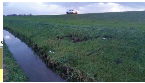
Figure 1.3: Slope instability of a inner slope levee (Evers, 2018, p. 26)
