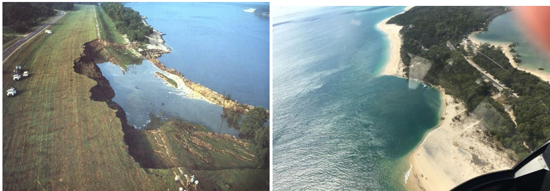
Figure 1. Damage to a river dike caused by a flow slide, from US Army Corps of Engineers, with the permission from Rogers, J.D. 2018 ( left ) [9]. A large collapse of beach at Inskip Point in Queensland due to a breaching event, with the permission from Rainbow Beach Helicopters Australia, 2019 ( right ) [10].
