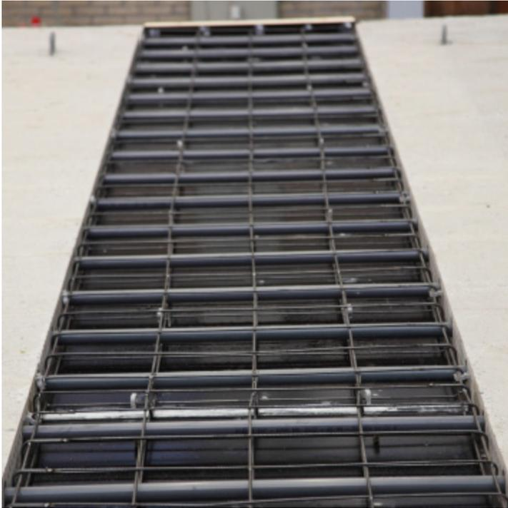
*Fig. B3-1 Ordinary steel reinforcement detailing of the transverse beams.*
