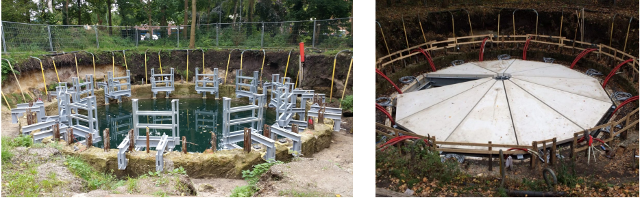
Figure 7.2: Construction of the real Ecovat system.
