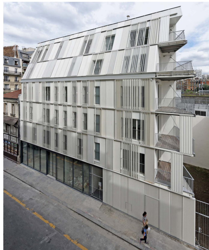
Aluminium louvers on social housing complex Paris - Dietmar Feichtinger Architects- David Boureau
