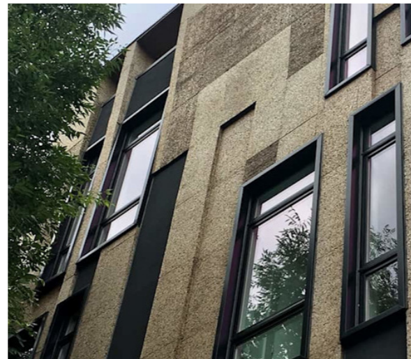
expanded cork facade-Amorim cork solutions
