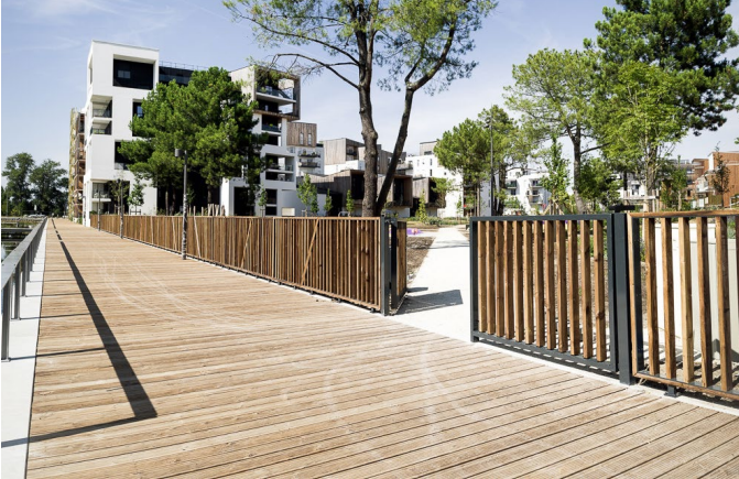
3.40 Eco-quartier Ginko Bouygues Immobilier | Bourdeaux, France
