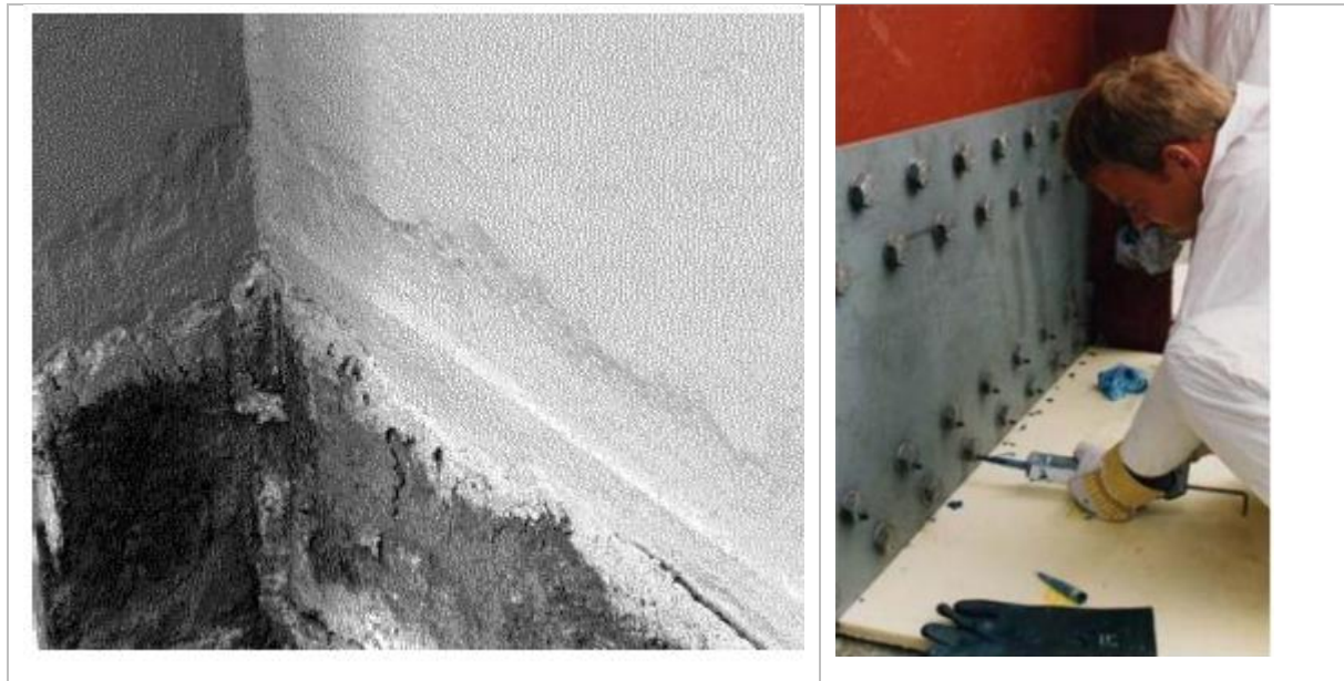
Figure 5 Corrosion of steel structure and subsequent repair with injection bolts [9]
