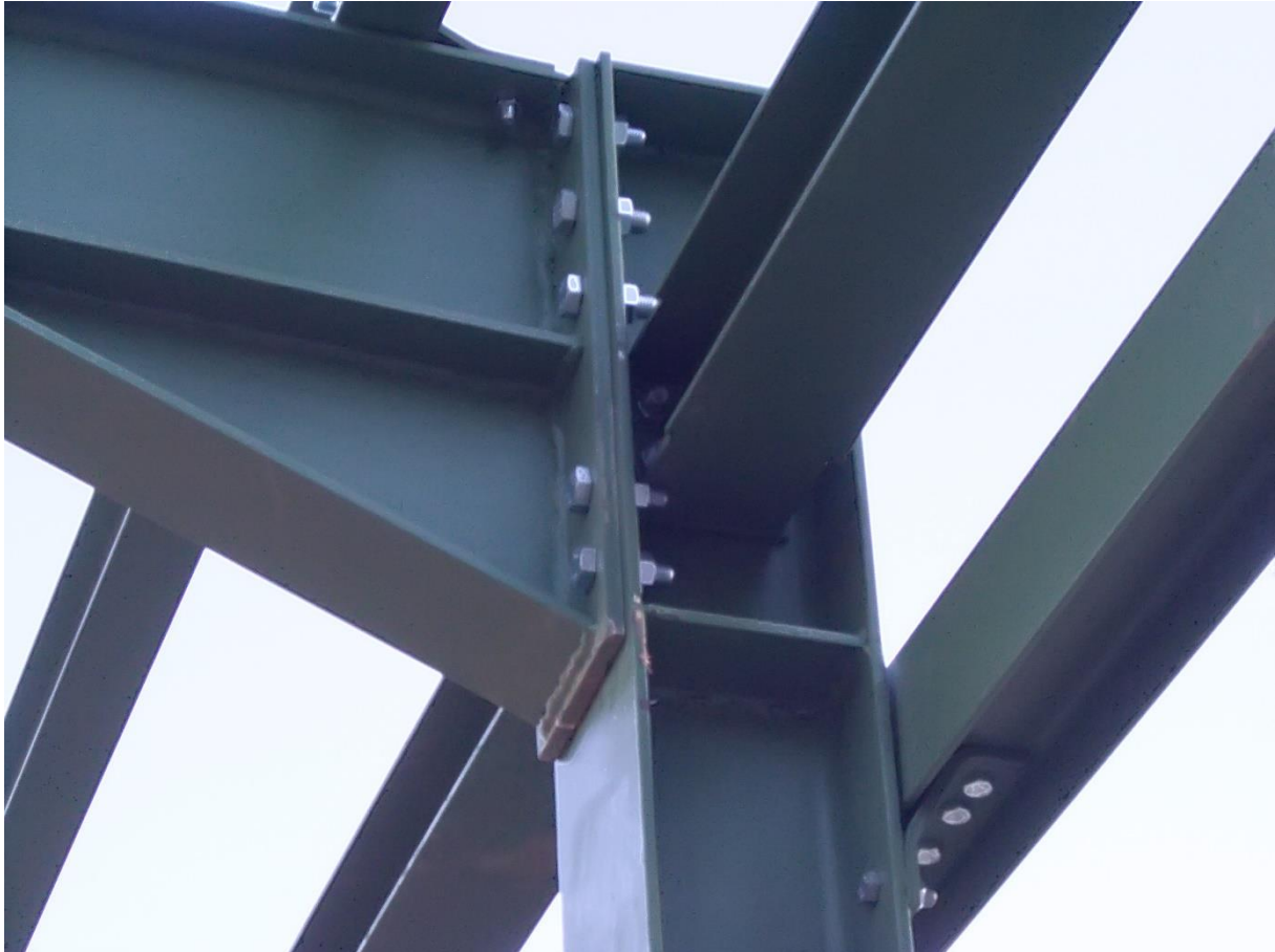
Figure 1 Example of bolted connection in steel structure [2]
