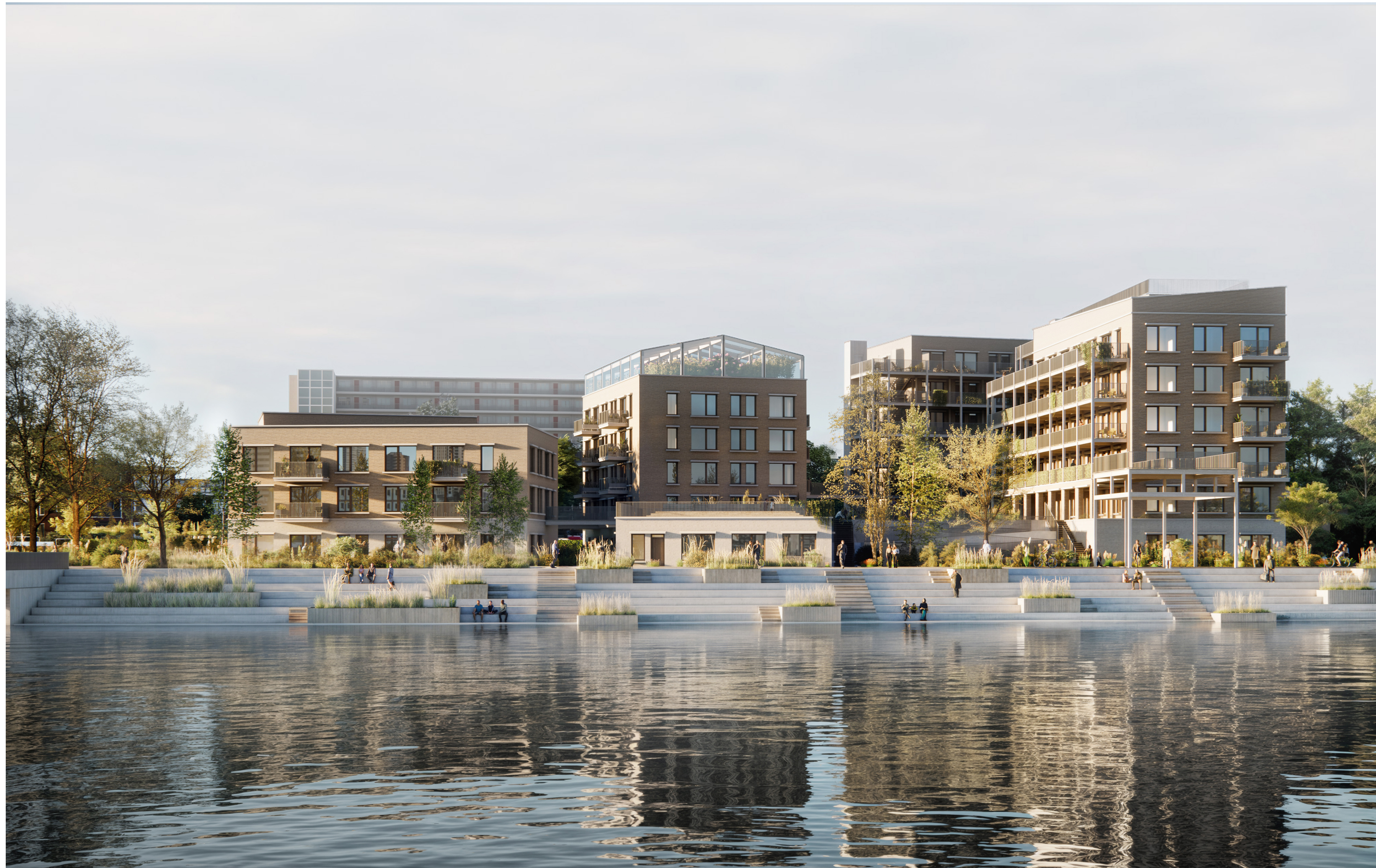
The housing ensemble viewed from the harbour
