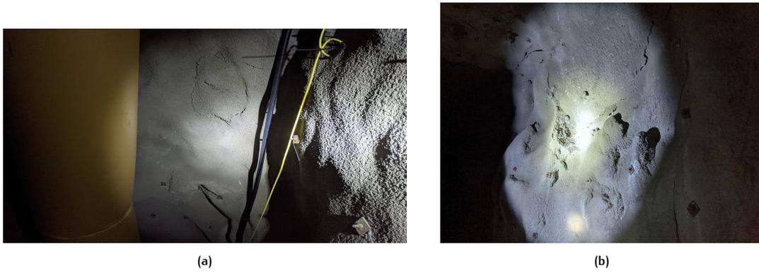
Figure 6.25: Shotcrete damage found in L62-H as result of convergence. (a) Shotcrete damage in the top right wall. (b) Shotcrete damage in the right wall.
