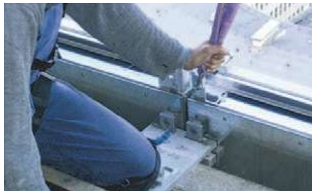
Fixing of a modular façade using HCW-ED Brackets on HTA-CE Cast-in channels
