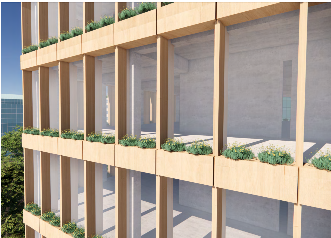
Render 12: Close-up rende composite timber facade Author's own work.
