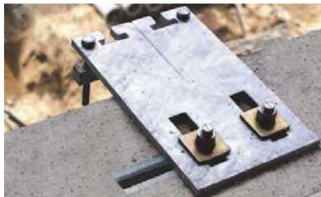
Typical curtain wall fixing with HTA-CE Cast-in channels
