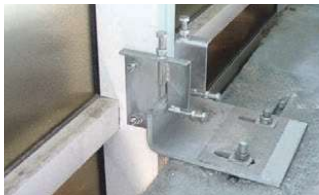
Fixing of a curtain wall system using HCW-B2 Brackets connected to HTA-CE Cast-in channels
