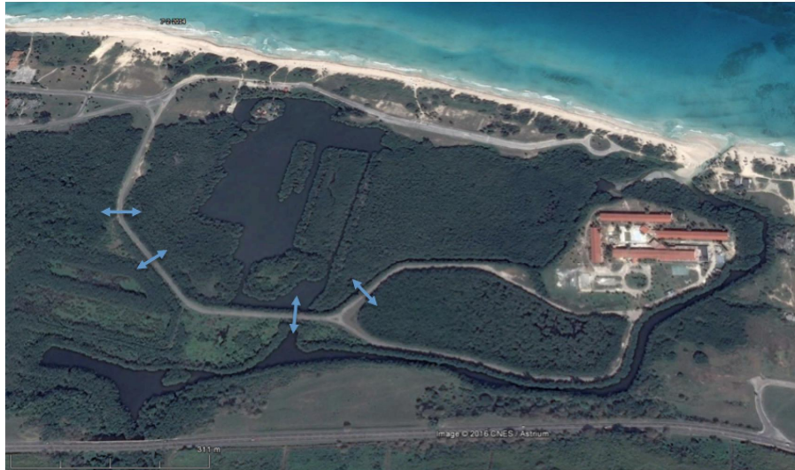
Figure 2.15: Locations of the culverts [26]
