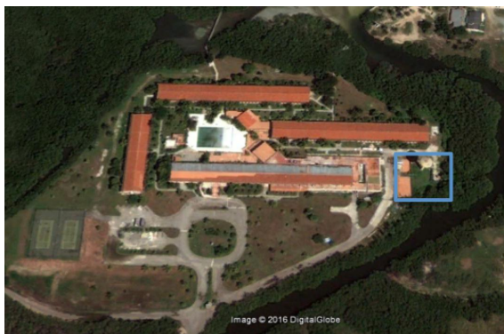
(a) Wall structure around the WWTP
