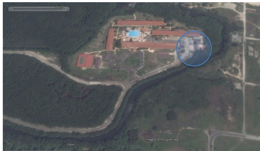
Figure 2.4: Aerial overview of the Blau Arenal Hotel and location of the new waste water treatment plant (blue circle), satellite image from 29-06-2015 [5]
