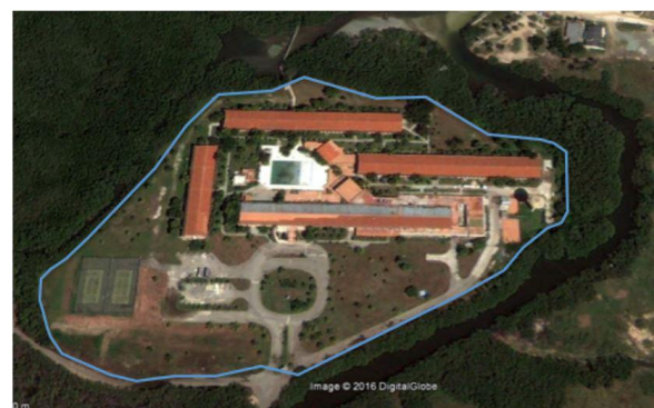
(b) Wall structure around the Blau Arenal Hotel and the WWTP
