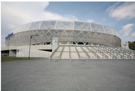
Figure 1.13: Allianz Stadium, Nice - France [31]
