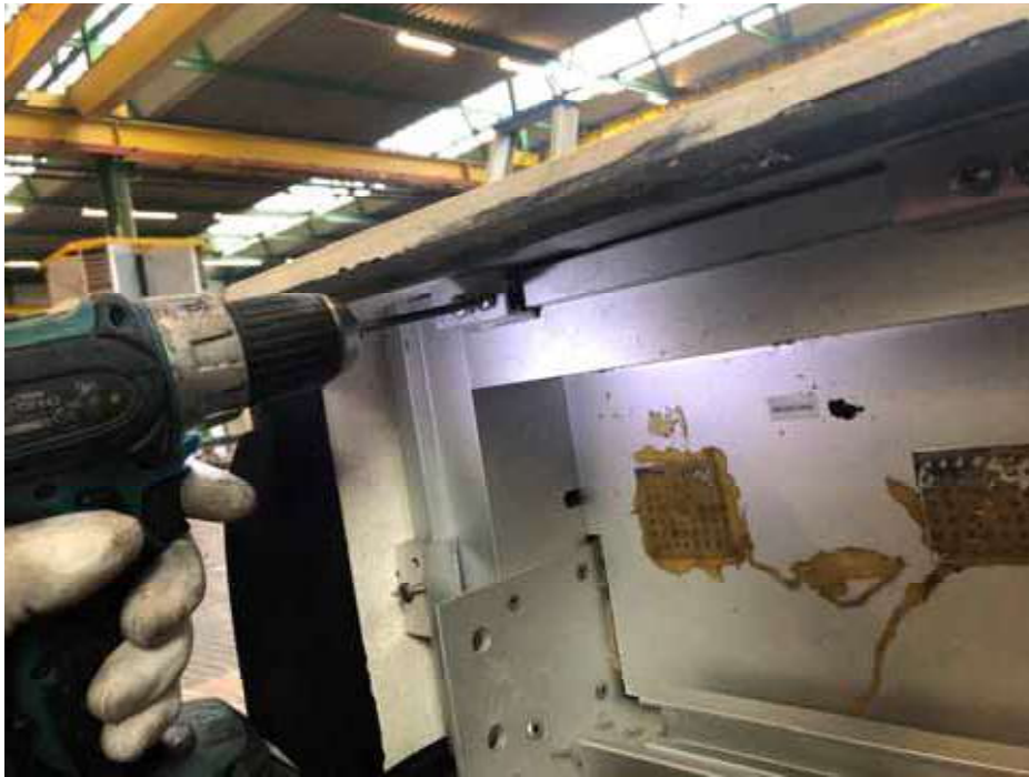
Step 1 – Removal of GRC elements
