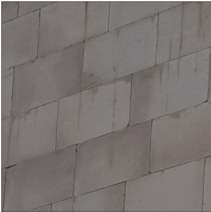
AAC masonry load bearing walls
