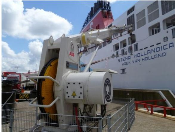
Figure 6.2: Aft - crane on shore with integrated cable reel in Hoek van Holland, image from [9]
