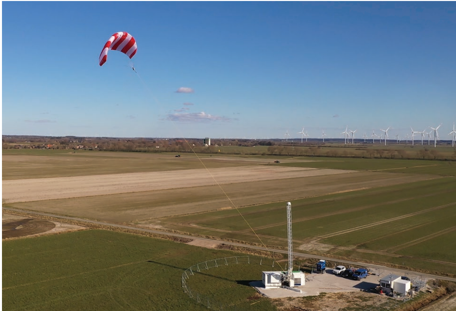
Figure 4.1. The studied test site, featuring a ground-generation airborne wind energy system with a soft-wing kite. In the background, one of the many nearby wind farms is visible (Courtesy of the SkySails Group).
