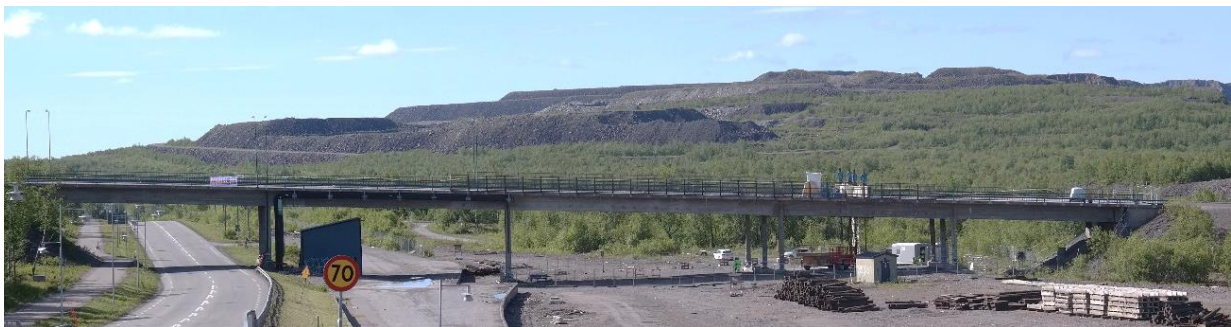
Figure 9 - View of the Kiruna bridge from north.
