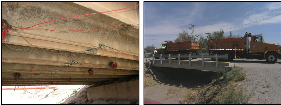
Figure 13 – Instrumentation and proof testing of Bridge No. 7701
