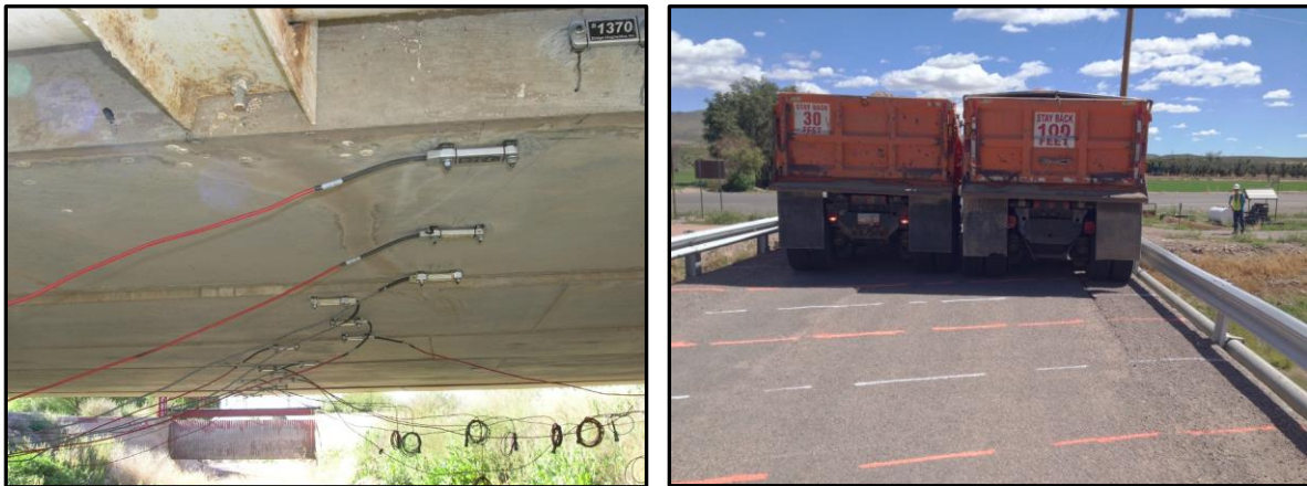
Figure 14 – Instrumentation and proof testing of Bridge No. 7722
