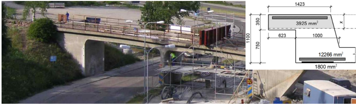
Figure 5 - The tested railway bridge in Örnköldsvik (Övik), Sweden, in a view from the West side showing the test setup. A cross-section is shown as an insert of one or the two beams with a height of 1,100 mm (3.6 ft) and a bottom reinforcement of 12,266 mm 2 (19sq.in.) steel bars and 1,800 mm 2 (2.8sq.in.) carbon fibre reinforced polyester (CFRP) bars. (100 mm = 3.9 in, 1000 mm 2 = 1.55 sq. in.).
