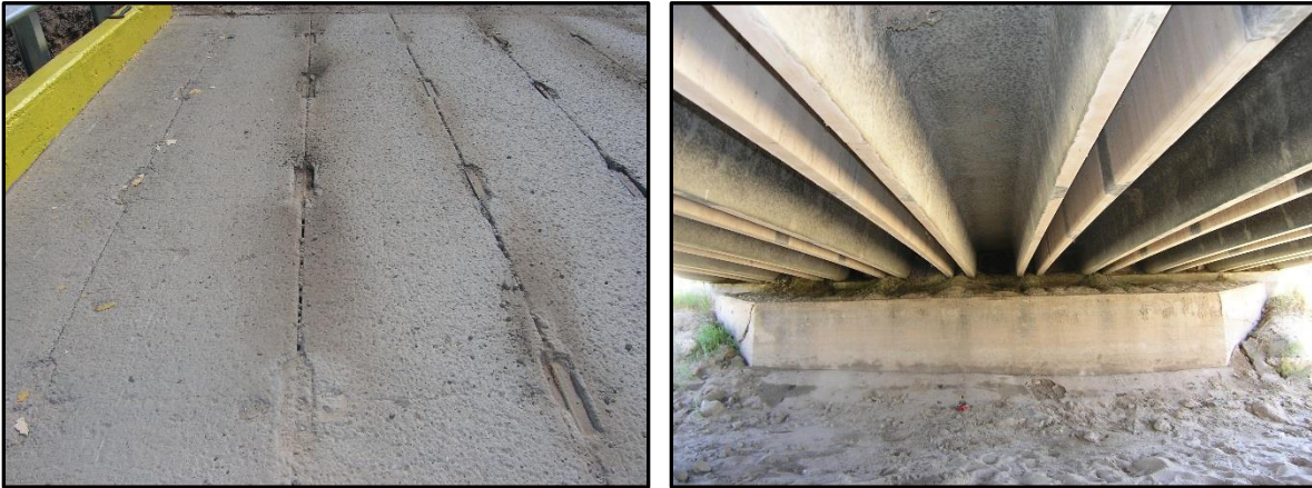
Figure 1 – Bridge No. 7701 (prestressed concrete double T-beam)
