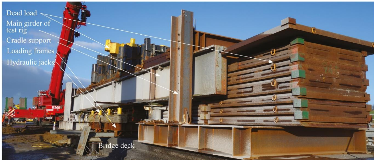
Figure 8 – Overview picture from testing performed on bridge #2
