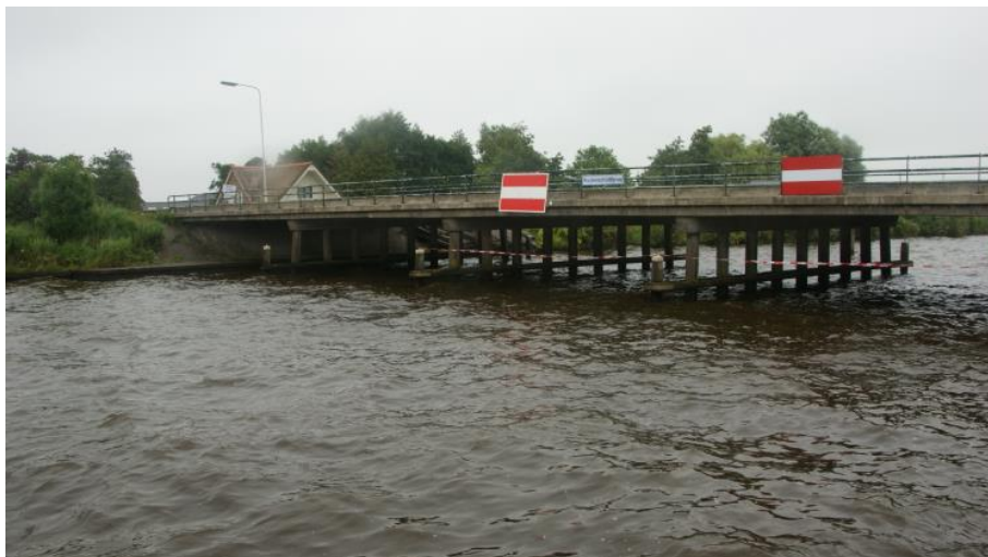
Figure 4 — Ruytenschildt Bridge in 2014.
