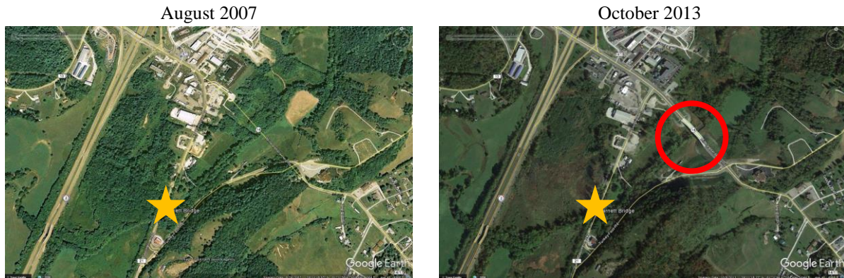
Figure 14 — Construction of the Bypass (Circled) Relative to Barnett Bridge (Starred)
