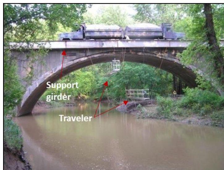
Figure 6 — Barnett Bridge under the 400k Load Stage
