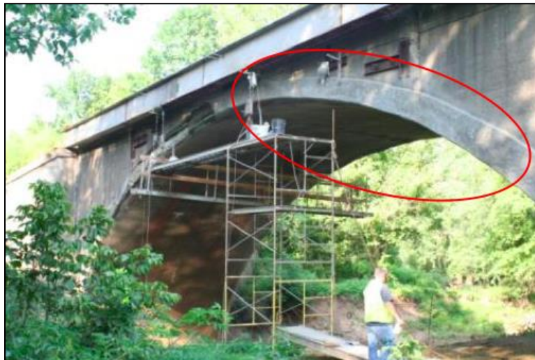
Figure 11 — Repair of the Arch Ring in Progress
