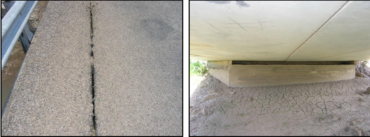
Figure 2 – Bridge No. 7722 (prestressed concrete box beam)
