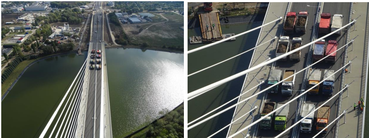
Figure 1. The application of proof load onto cable-stayed bridge on Wisłok river (phot. K.Wilde).
