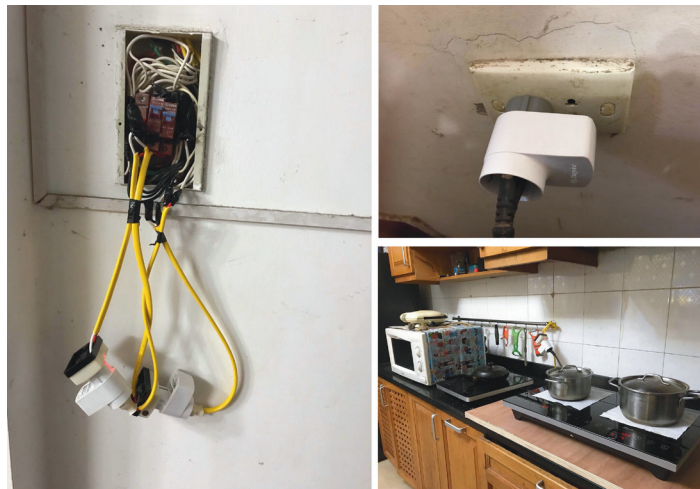
FIG. 7.2 Plug-wise unit installed for energy measurement
