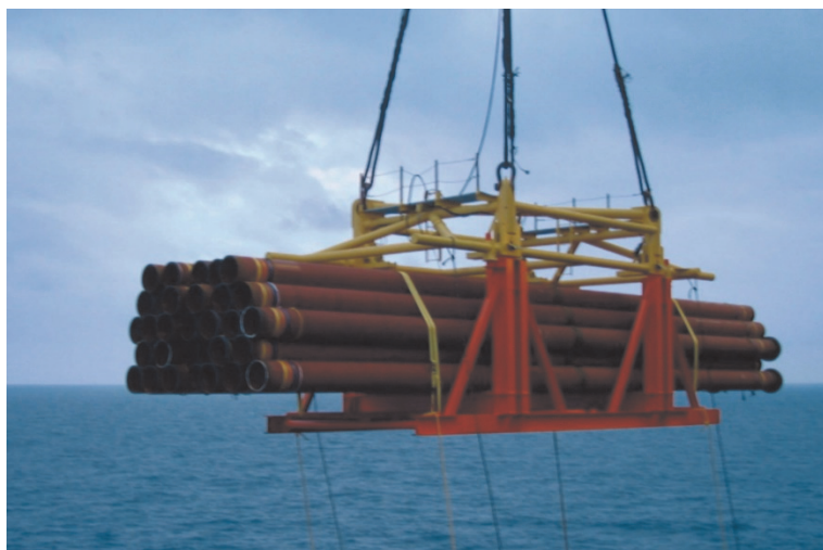
Figure 2-4 Riser pipes (double joints).
