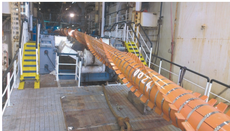
Figure 2-16 Installation of deep water riser with VIV suppressing strakes. Installation of an OD 456 mm SCR with S-lay method on a dynamically positioned pipe-lay vessel in approximately 1300 m water depth. The VIV suppressing strakes are clamped on the pipe with stainless steel straps before the pipe enters the water. Source: Allseas (2019).
