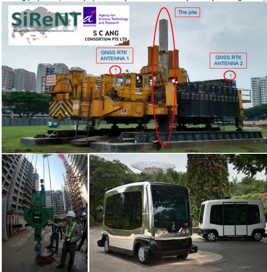
Figure 1.5: Applications using SiReNT; the semi-automated piling system (top), the semi-automated tower crane system (bottom left), and autonomous vehicles at Gardens by the Bay (bottom right). Source: SLA
