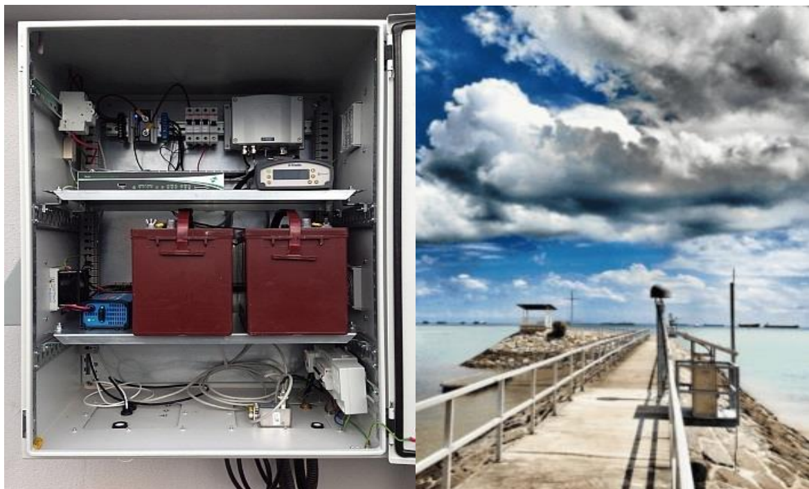
Figure 1.4: An example of the SiReNT CORS set-up; a weather-proof steel cabinet housing, containing Trimble NetR8/Trimble NetR9 GNSS receivers, modem/routers and back-up batteries in case of a power outage (left) and the antenna (right). Source: SLA.
