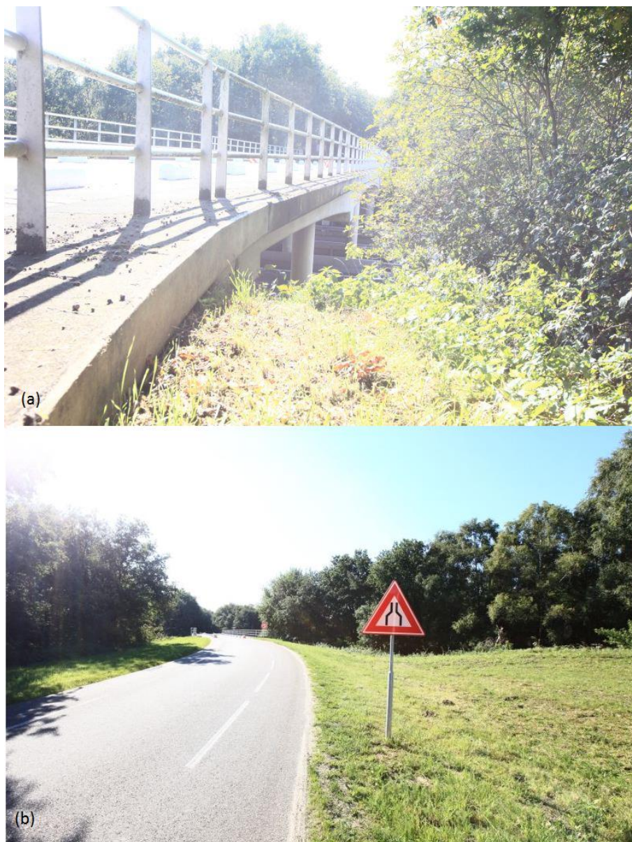
Figure 6: Viaduct De Beek (a) side view; (b) traffic restriction.
