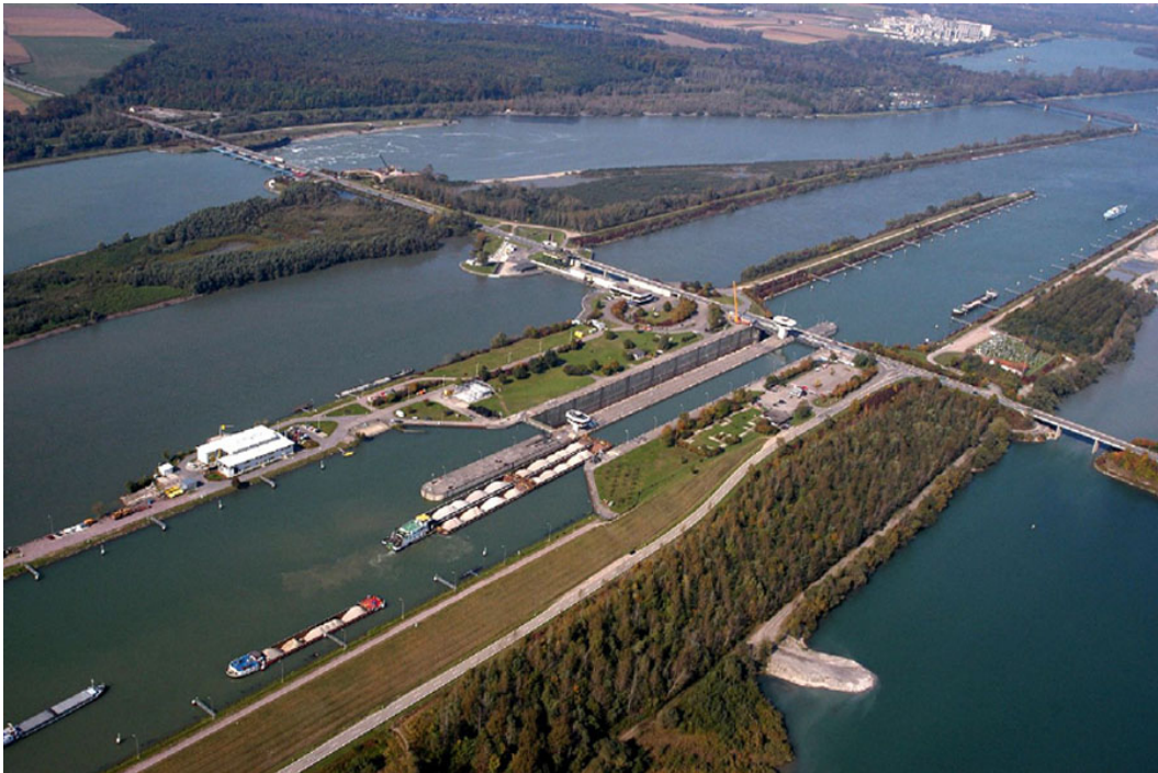
Weir at Iffezheim, Rhine river, southern Germany
