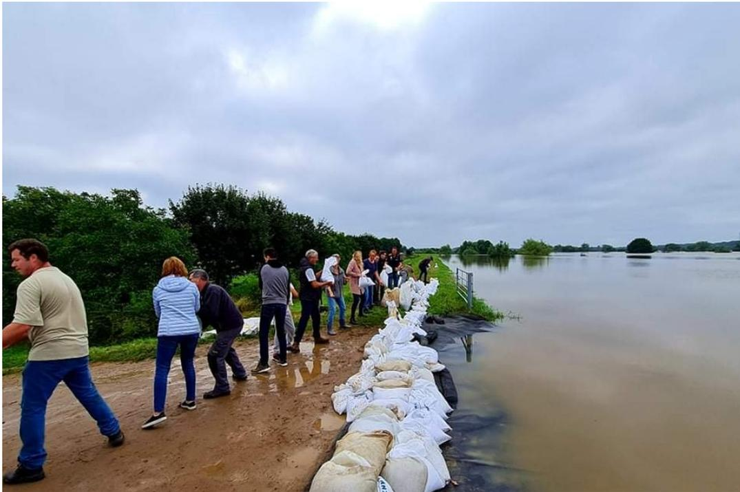
**Figure 1.1:** Reinforcement of the dike with sandbags near Buggenum (De Limburger, 2021)
