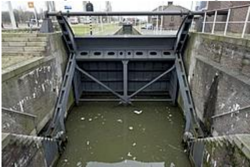
Figure 62 Tainter gate, without counterweight, www.debinnenvaart.nl
