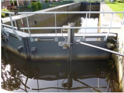
Figure 15 Mitre gate, source:www.rolanco.nl
