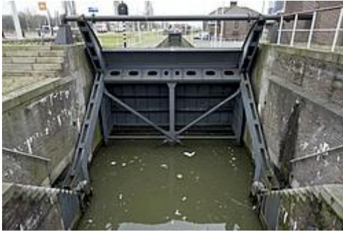
Figure 13 Tainter gate, without counterweight, www.debinnenvaart.nl
