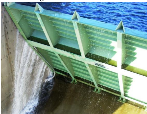
Figure 63 Tumbler gate (not used for a navigational lock at the picture) www.vortexhydradams.com
