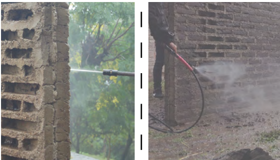
bricks were pushed out with pressure washers
