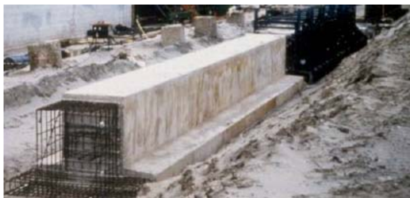
Figure 5.6: Landward crane girder – under construction
