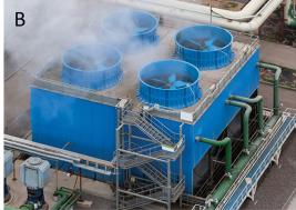
**Figure 1.1.** (A) 122-meter-tall natural draft cooling tower (Tim Reckmann) and (B) 10-meter-tall induced draft counterflow cooling tower (https://water.aecsi.us).
