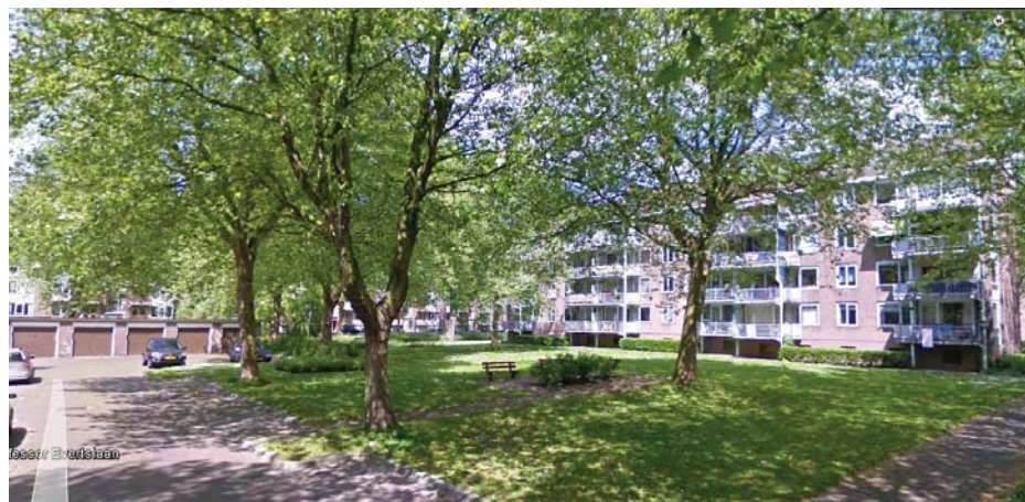
(2) Inner courtyard with grass and benches, garage boxes at the end of the access street
