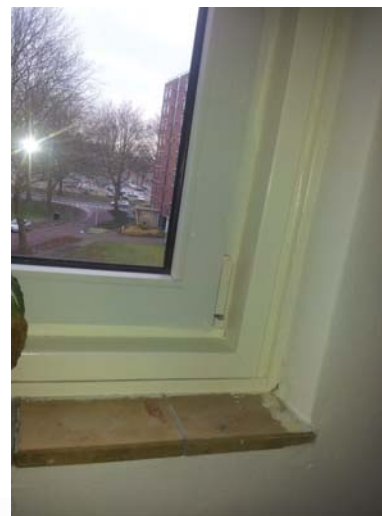
New window frame - plastic window frame and wooden frame
