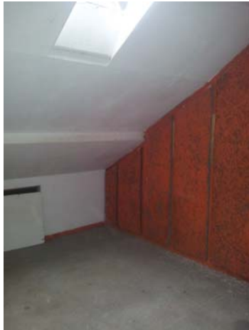
Room made in the attic
