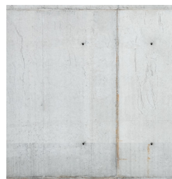
Off-form concrete wall
