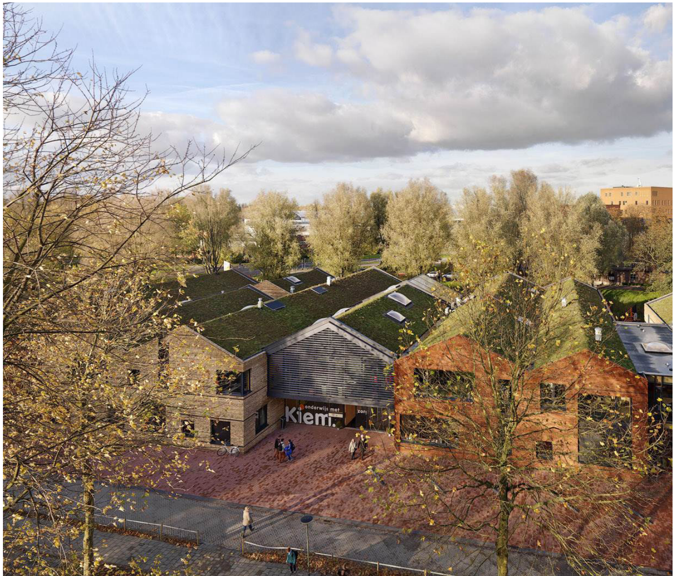
Figure 38 Exterior view (Kiem Special Care school)
