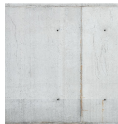
Off-form concrete wall
