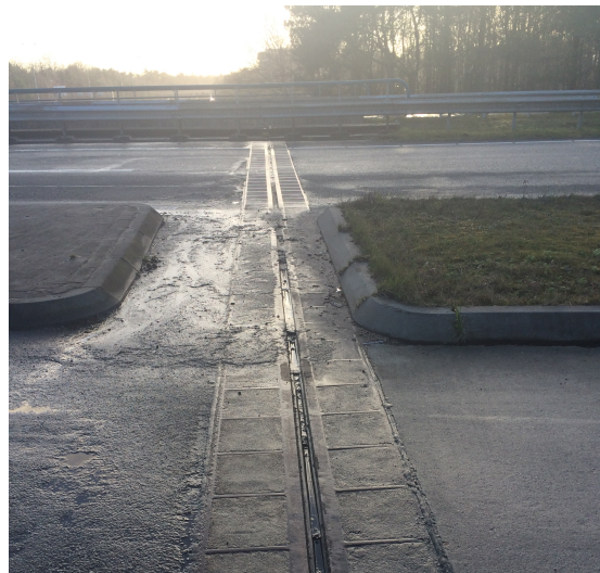
Figure 4: A picture of an expansion joint of type SN ESV-R1, located at the bridge "Zandbergen" (N238).
