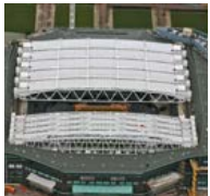
Wimbledon Stadium Roof, Capita Symonds
