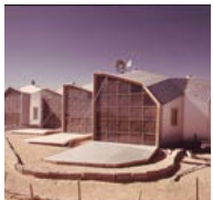
Baer House, Steve Baer
